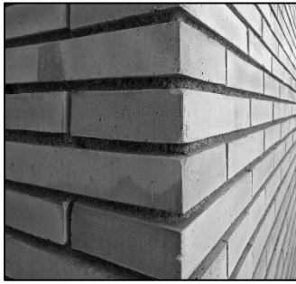
FIGURE 8: Wall masonry corner wrapping
