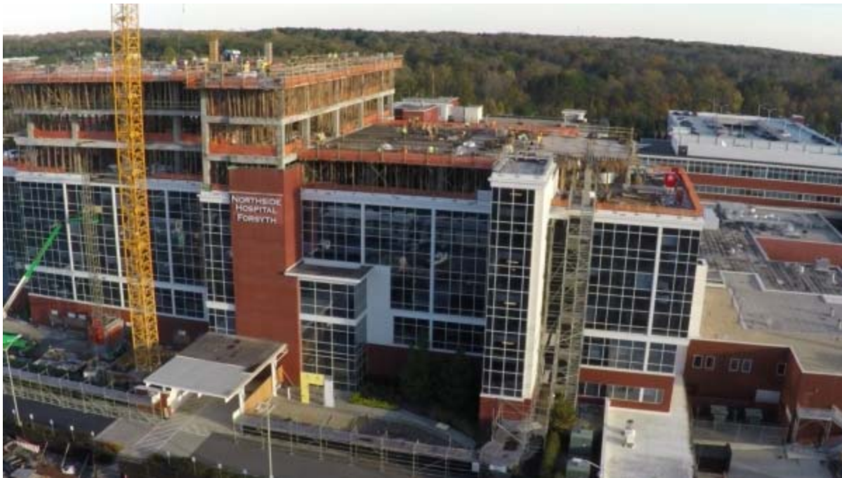
Figure 5: Northside Hospital – Forsyth Construction (myforsyth.com, 2016)
