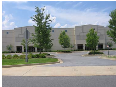
Vacant Publix warehouse/distribution building - Cabot Business Park
