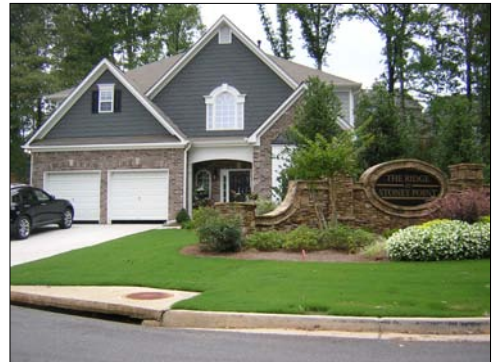
Example of residential style in the area
