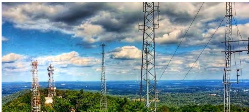
Radio Towers on top of Sawnee Mountain
